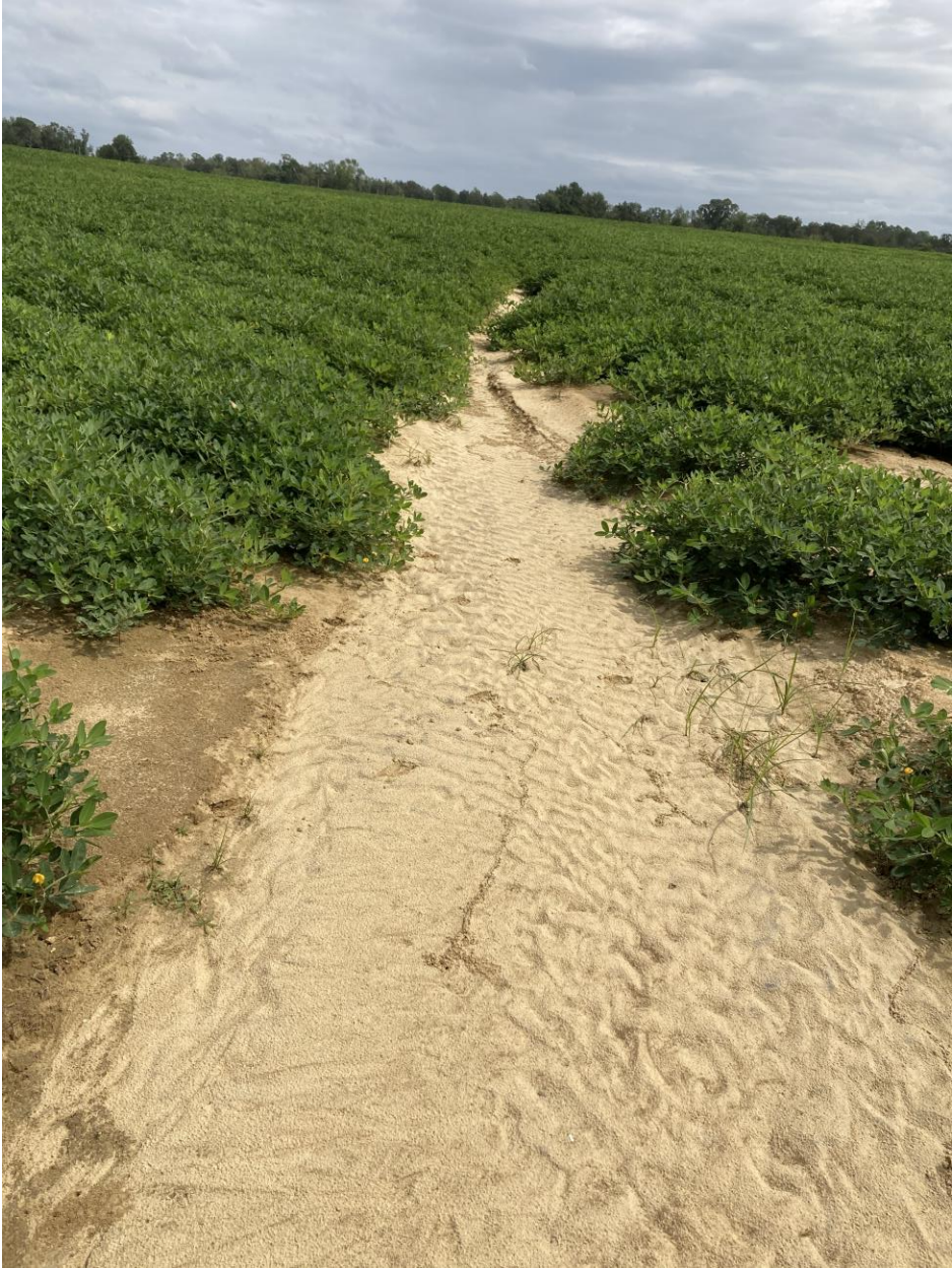
Water erosion near Whiteville, NC
